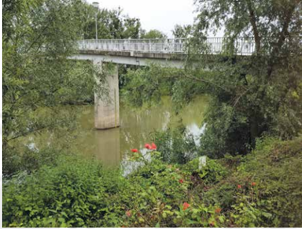
Martin-Roth-Brücke in Erfelden
